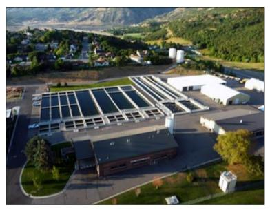
**Coagulation** and **flocculation** is the first stage in water treatment. The goal of this stage is to bind up the suspended particles included in the raw water by adding a coagulant to the raw water as it first enters the water treatment plant. Floc, which is a tuft-like aggregate, is produced from the mixing of the coagulant in the raw water. This process is called flocculation. Over time, as more suspended matter is bound, the smaller aggregates of floc become larger particles of floc.
